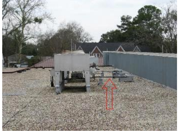
PHNS: Active Leak Area Hallway in front of Data Processing
