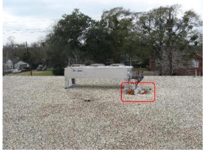
Data Processing Area Light panel in right center corner
