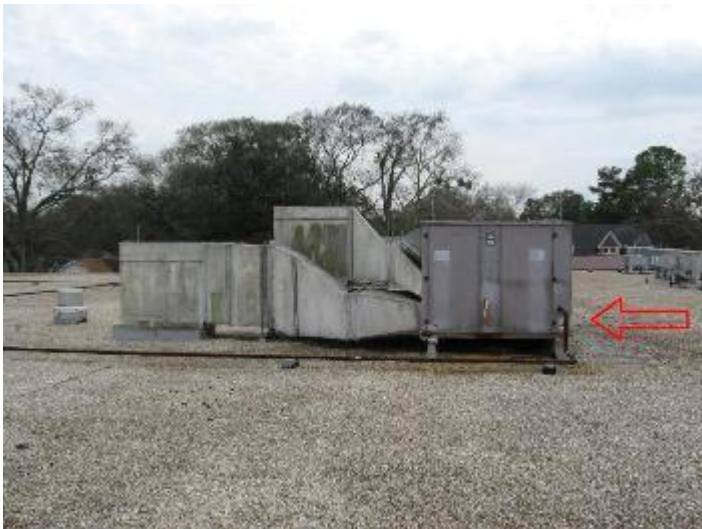
PHNS: Active Leak Area Middle of Conference Room 1
